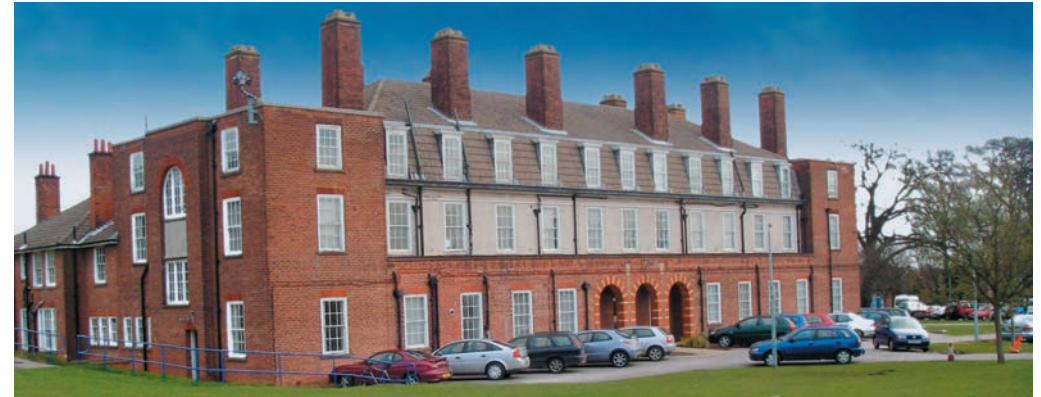
Finance Building: demolished mid 2017
