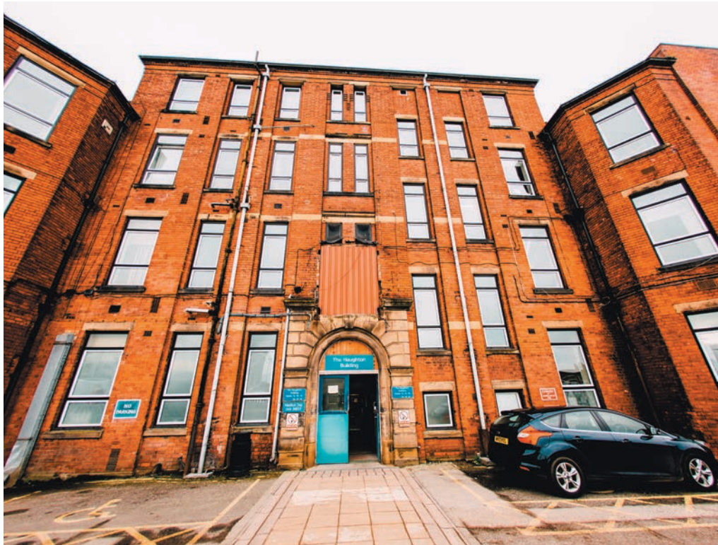
Haughton Building (West): to be demolished mid 2017
